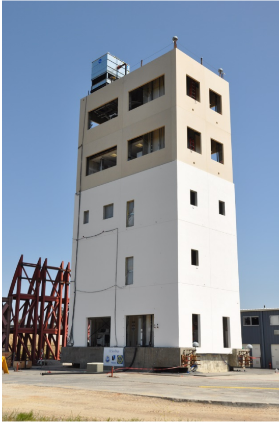
Figure 3–3. UC San Diego tested this full-scale building, outfitted with nonstructural components such as an intensive care unit, a surgery suite, piping, ductwork, fire barriers, and a working elevator, on its NEES shake table. © 2013 Image Courtesy of Tara Hutchinson.
